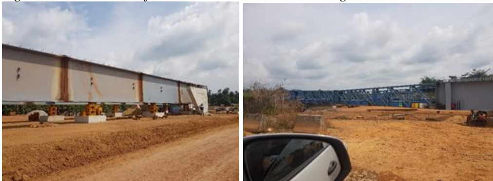
Figure 10: Fabrication of steel beams on site and launching nose secured
