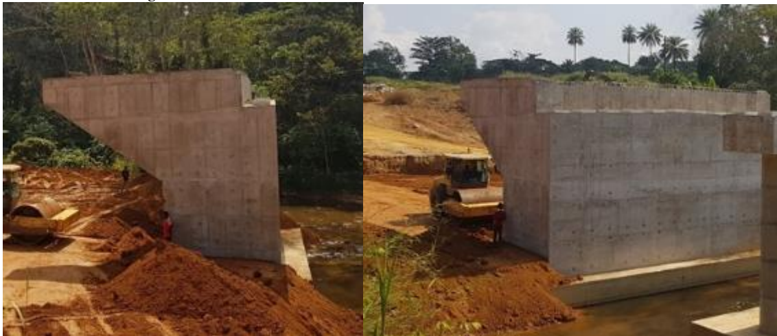
Figure 16: Cantilever solid wall abutment
