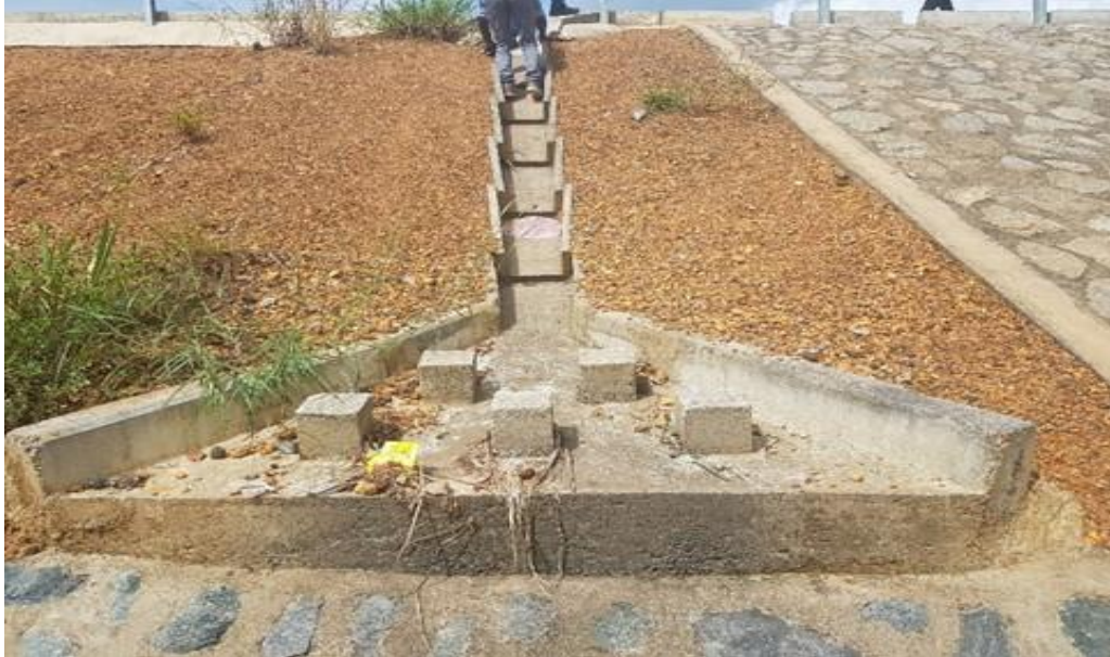
Figure 20: Typical down chute
