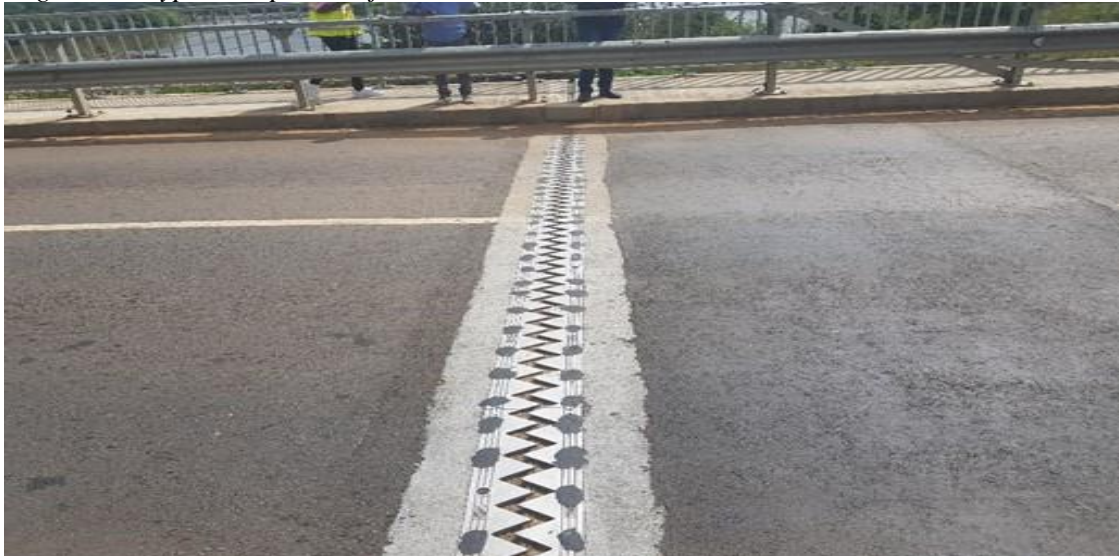
Figure 17: Typical Expansion joint
