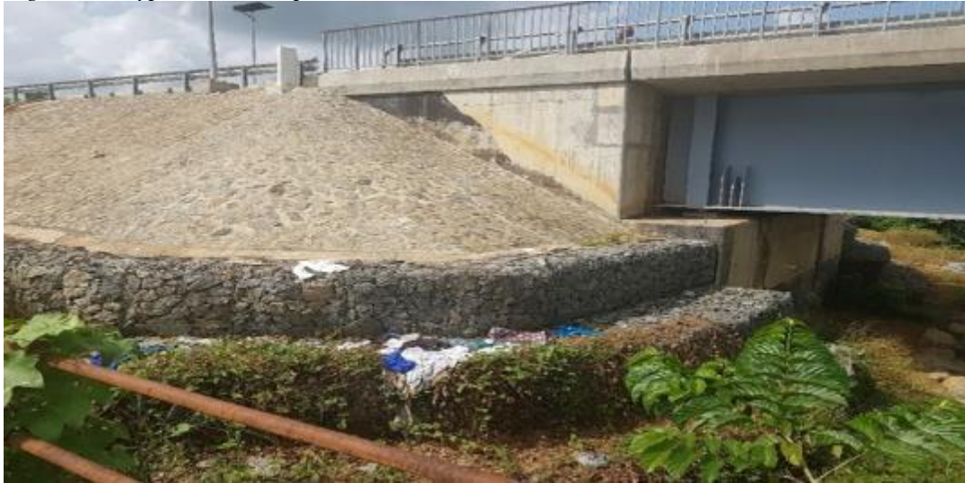
Figure 18: Typical erosion protection at Abutment
