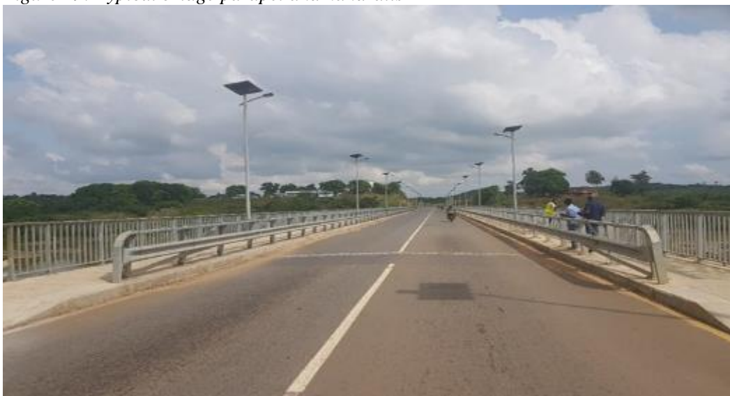
Figure 19: Typical bridge parapet and handrails
