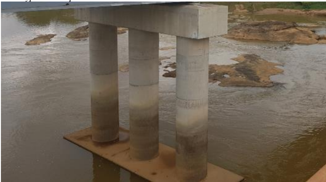
Figure 14: Typical Multiple Circular Columns Pier
