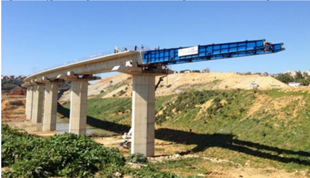
Figure 13: Typical bridge under construction using Incremental launching method
