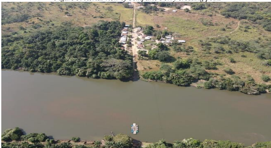
Figure 5: Aerial view of Tomparie Ferry crossing point
