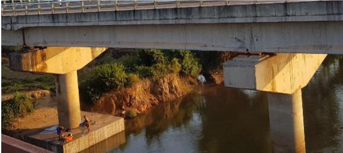
Figure 15: Single column with hammerhead Pier
