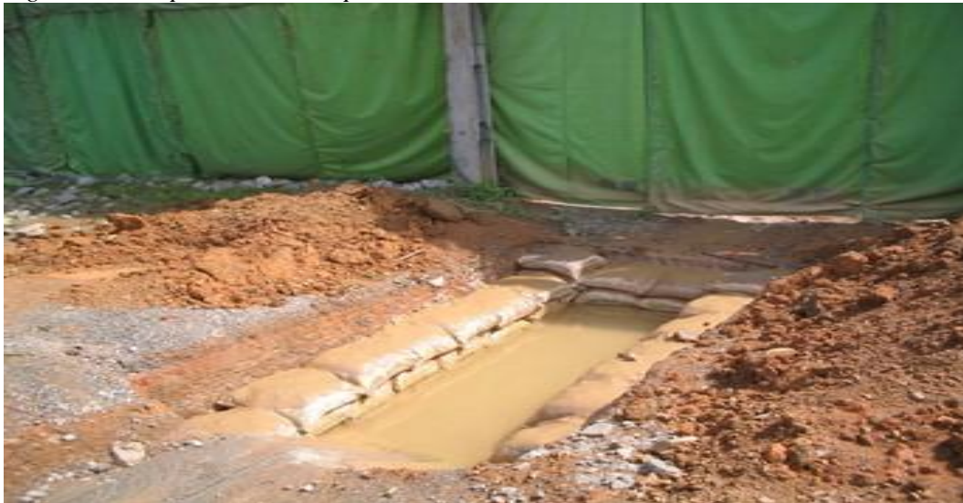
Figure 64: Sample silt removal ponds
